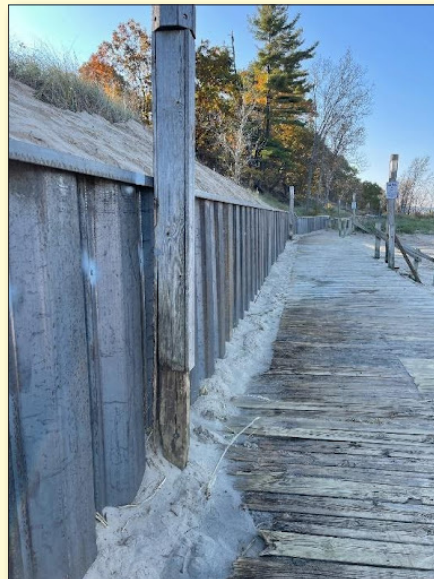
New retaining wall along the south boardwalk
